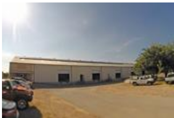
Caption: The fact that GECKO's facility is run largely on solar power is a testament to its dedication to operating in an environmentally sound manner. The company is also in the process of putting in a rainwater collection system to conserve water used in the stone fabrication process.
